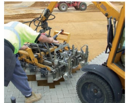
HVZ herring bone 45° - the ideal solution for bigger areas of herring bone pattern. This type of clamp handles 45° packed layers of stones and allows an installation without filling gaps by adding stones.
